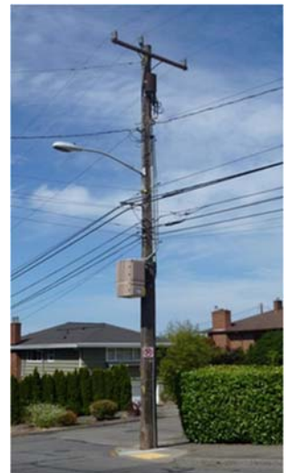
Example of a 5G antenna installed on a utility pole
