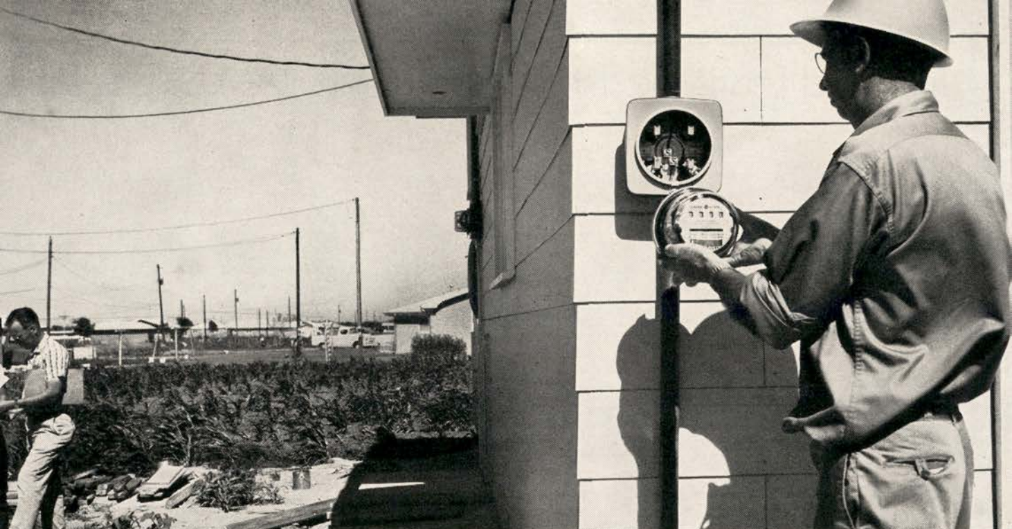
Electrician Otto Johnson installs General Electric I-55-S single-phase meter in General Electric S-1 square socket. Site is an all-electric home near North Platte, Nebraska—one of Dawson County Public Power District's 6,500 General Electric meter installations.
