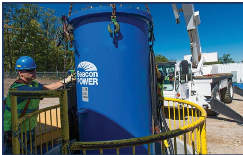
Flywheel energy storage technology installation at Chugach Electric Association
