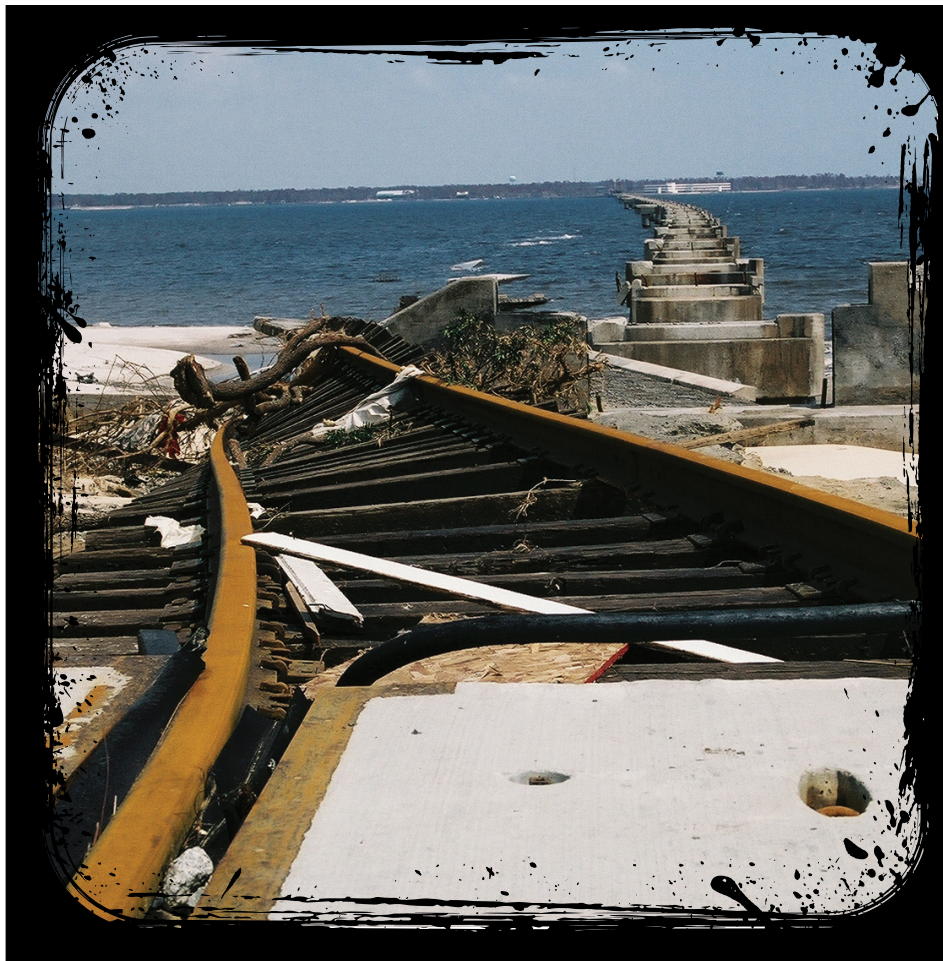
Mississippi's Bay St. Louis rail bridge sustained heavy damage from Katrina, but the support piers withstood the storm and were used to rebuild the structure.
