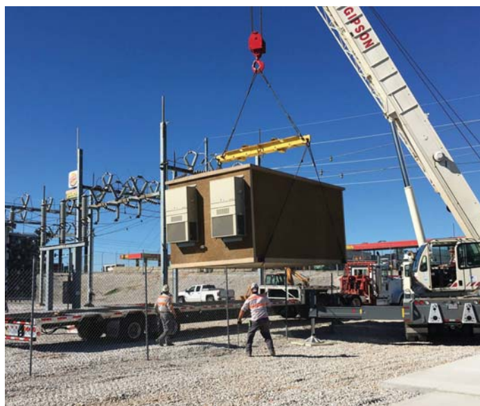
Crews install a telecommunications hut at a substation as part of Diamond State Networks’ middle mile broadband system.
