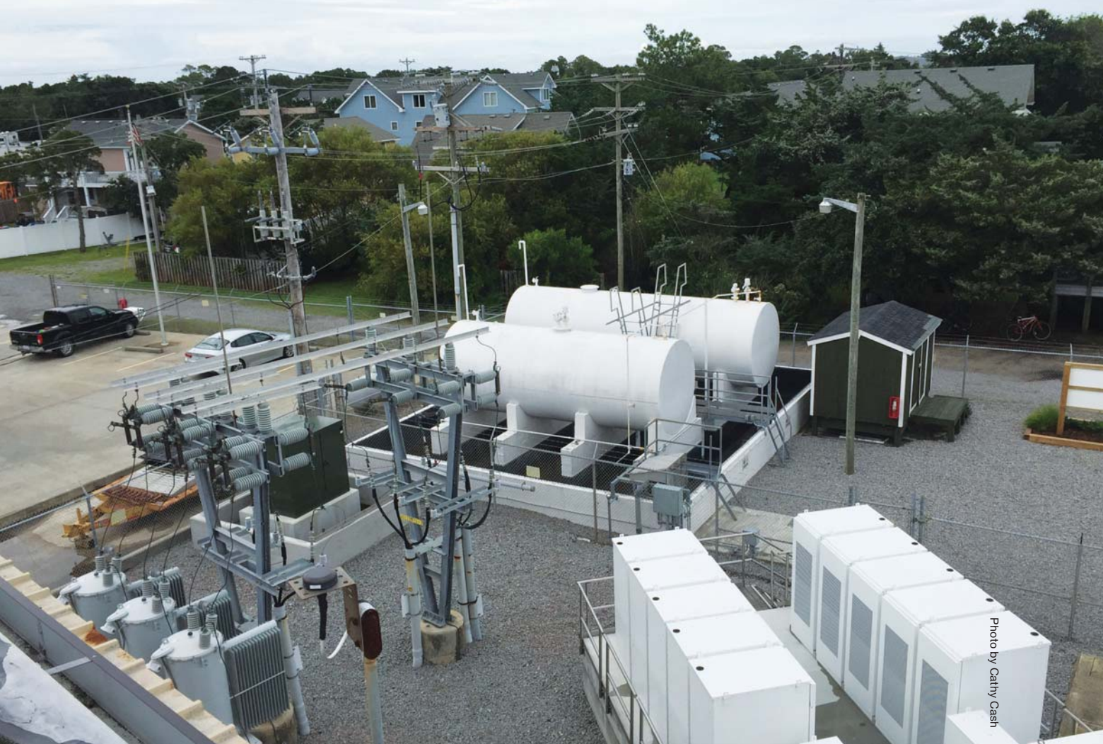
North Carolina EMC's microgrid campus on Ocracoke Island includes diesel generators, battery storage, and solar generation.
