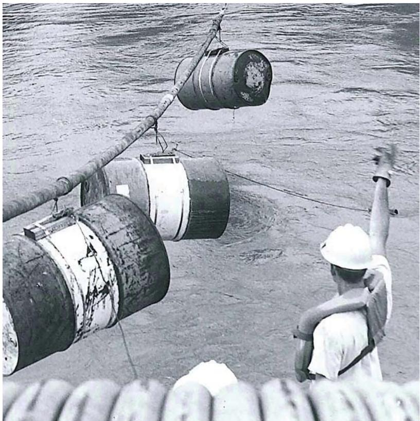
Weighted barrels helped lay the Hancock-Wood Electric power cable that stretches along the bottom of Lake Erie to Ohio’s Kelleys Island.
