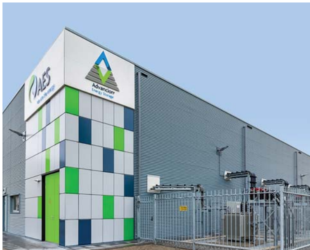
An AES battery storage facility
