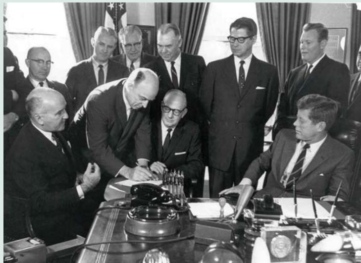
NRECA President Clyde Ellis (center-left) signs the first electrification contract with USAID as President Kennedy (seated right) looks on.
