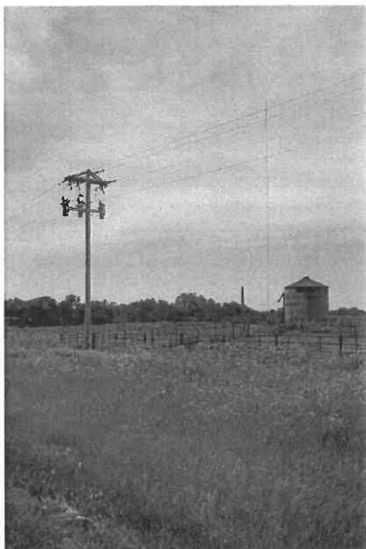
A utility pole (left) and cell tower outfitted with “fixed wireless” internet antennas (right) stand beyond a farm in rural Iconium, Iowa
