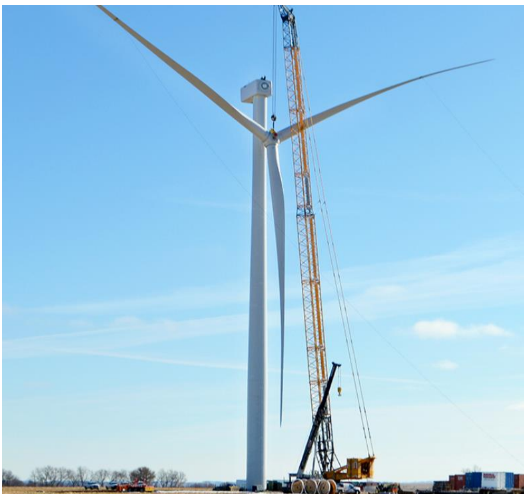
Image 1: Cuming County Public Power District purchases electricity from this 2.5 MW GE wind turbine with an 89-meter hub height and a 127-meter rotor diameter.
