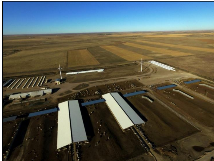
Figure 3. Heritage Dairy's Wind Turbines in Y-W Electric Association, Inc. Service Area.
