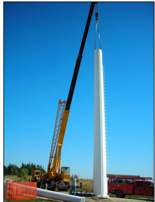
Figure 6: Medium-sized wind turbine tower installation.
