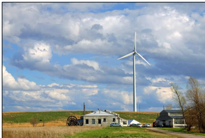
Figure 4. Abandoned Crown I Coal Mine buildings at the GobNob wind turbine site. Courtesy of RECC.
