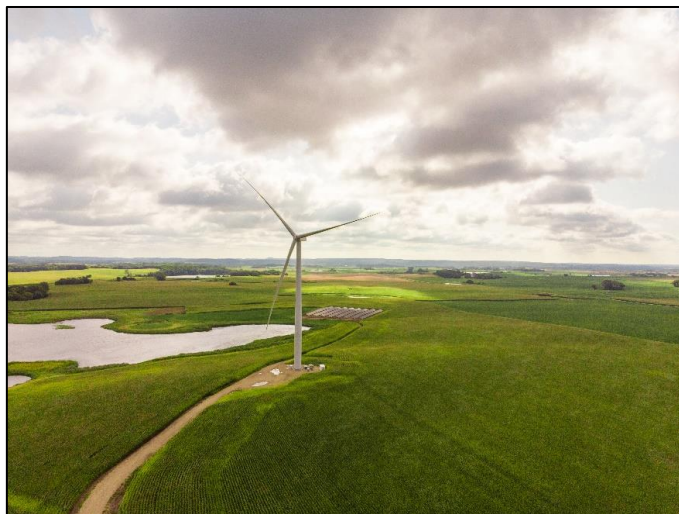
Figure 6. Lake Region's Wind-Solar Hybrid Project, located on a member's farmland. Courtesy of Lake Region Electric Cooperative.
