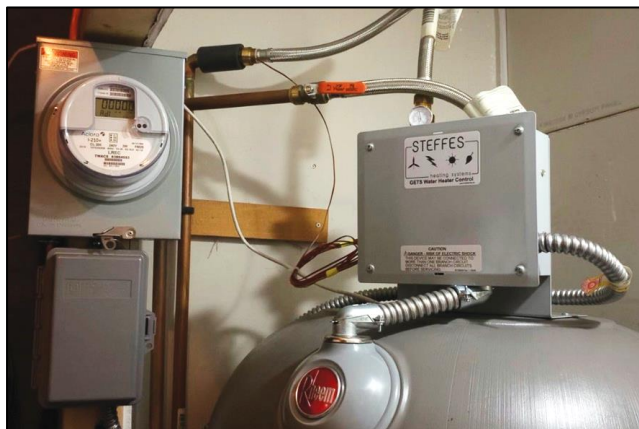
Figure 4. Steffes GETS controller on a member's water heater. Courtesy of Lake Region Electric Cooperative.
