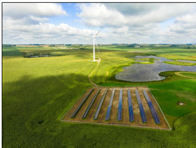
Figure 2. Lake Region's 2 MW Wind-Solar Hybrid Project. Courtesy of Lake Region Electric Cooperative.
