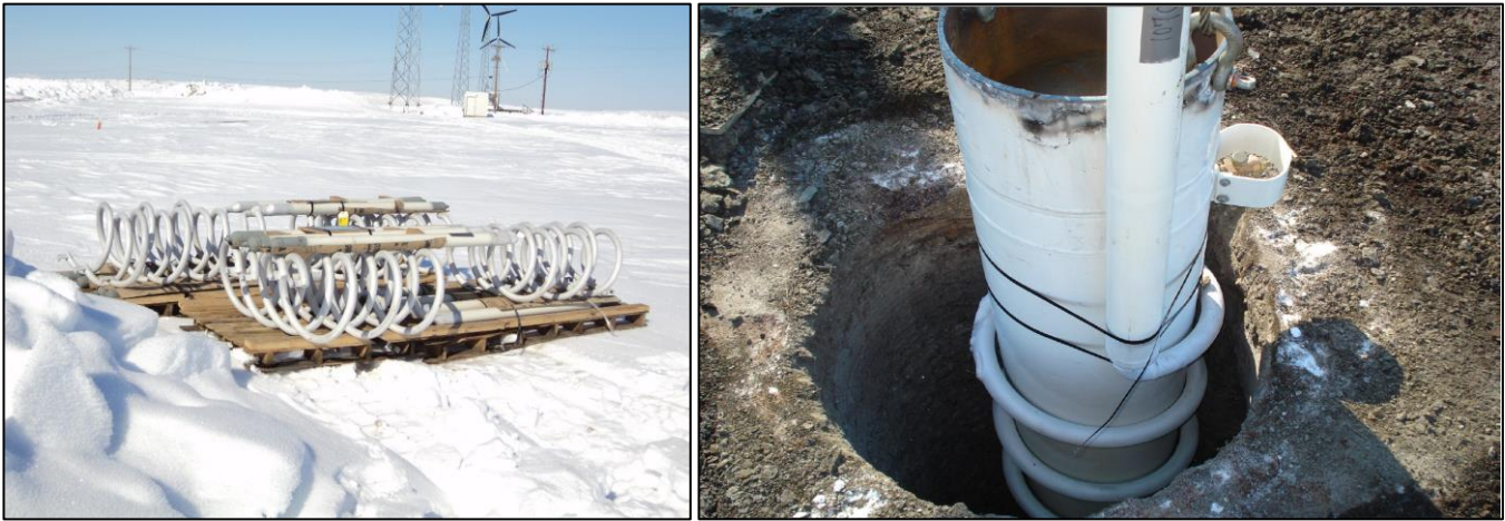
Figure 5. Thermal siphons to be installed as part of freeze-back pilings, and freeze-back piling installation. Courtesy of Kotzebue Electric Association.
