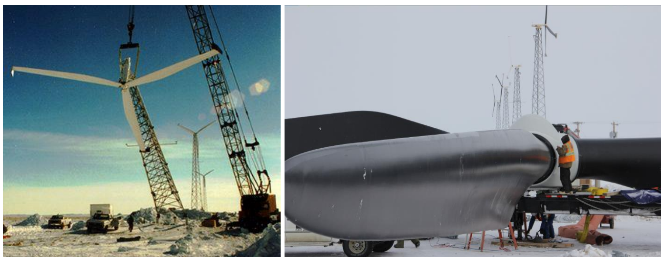
Figure 2. Wind turbine installations. Courtesy of Kotzebue Electric Association.
