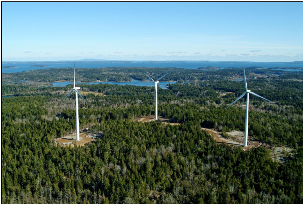
Figure 2. Fox Islands Wind Turbines.
