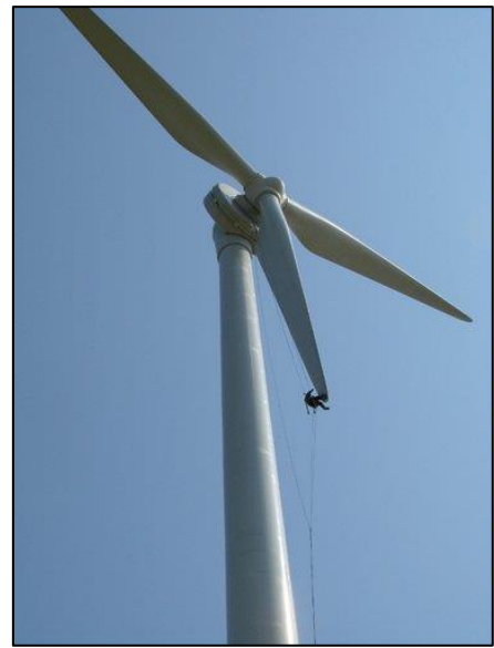
Figure 6. Technician repairs lightning damage to Pigeon Creek Wind Turbine blade tip. Courtesy of AEC.
