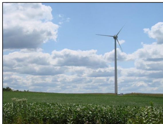
Figure 2. Pigeon Creek Wind Turbine. Courtesy of AEC.
