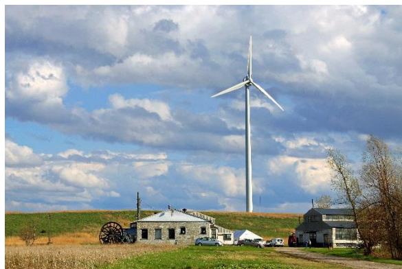
Abandoned coal mine buildings at the GobNob wind site. Credit: Rural Electric Convenience Cooperative
