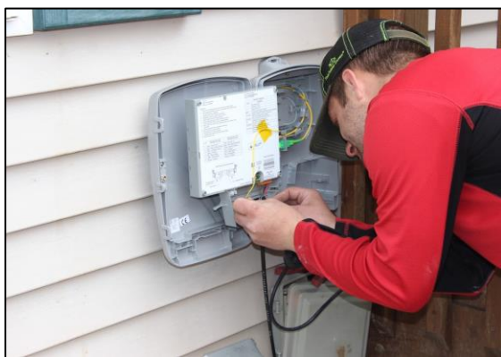
Figure 1. MEC technician installing a fiber drop. Figure 2. Checking wireless signal strength in a member's home. Photos courtesy of MEC.
