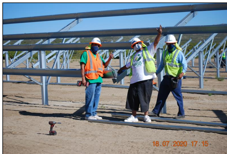
Figure 6: Anza Electric team working on the Santa Rosa Solar Project (Courtesy of Anza Electric)
