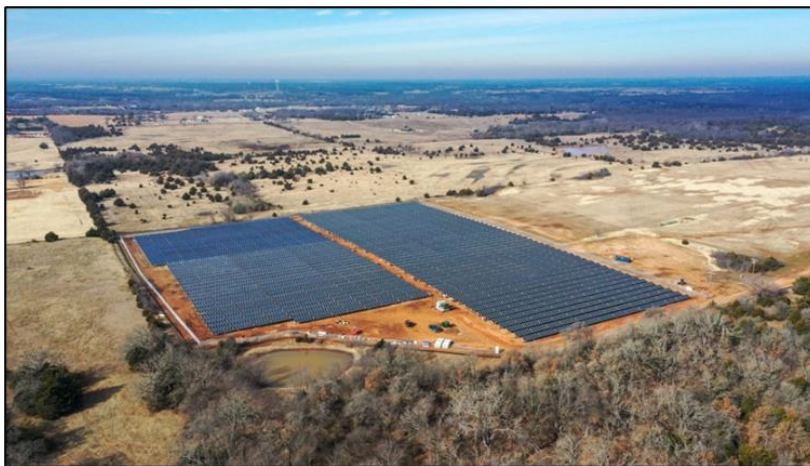
Figure 4: Oklahoma Electric Cooperative and Norman Public Schools Solar Array.
