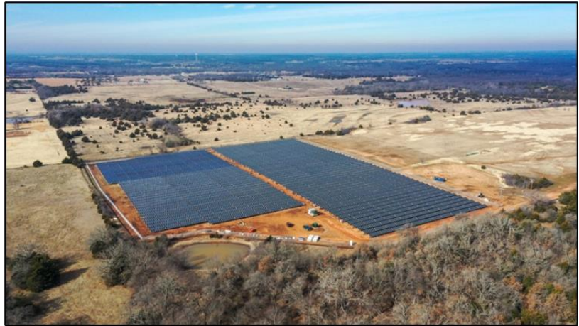
Figure 3: OEC and Norman Public Schools Solar Array (Image courtesy of Oklahoma Electric Cooperative)
