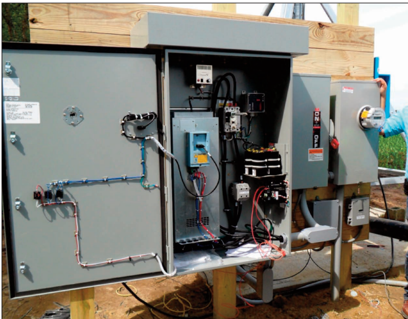
FIGURE 1: A VFD System Installation. Source: Delaware Electric Cooperative
