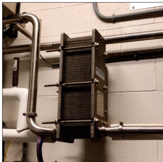
FIGURE 2: Kentland Flate Plate Milk Pre-cooler
