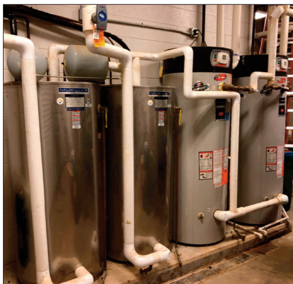
FIGURE 3: VT Preheater and Primary Heater Installation
