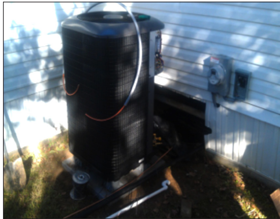
Figure 2: The outdoor unit of a new heat pump installed in a manufactured home
