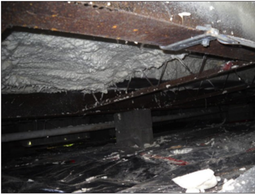
FIGURE 3: Spray foam installed between floor joists under a manufactured home. Photo courtesy of Buckeye Power
