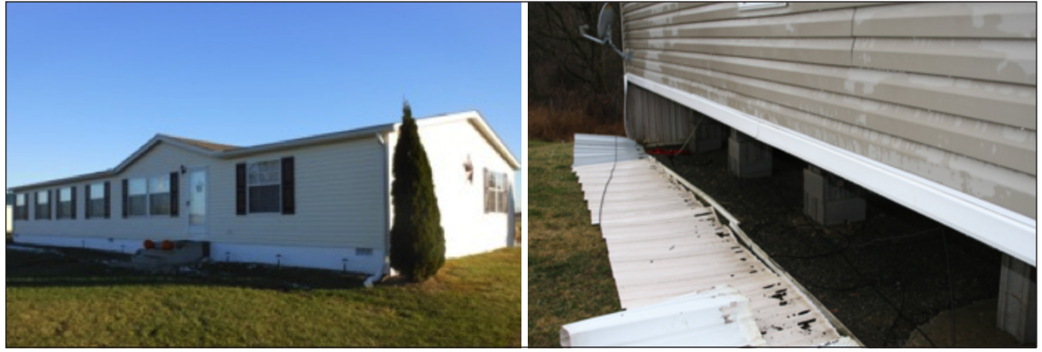
FIGURE 1: Manufactured homes may be sited on permanent foundations (left) or on blocks with protective skirting (right). Photos courtesy of Buckeye Power
