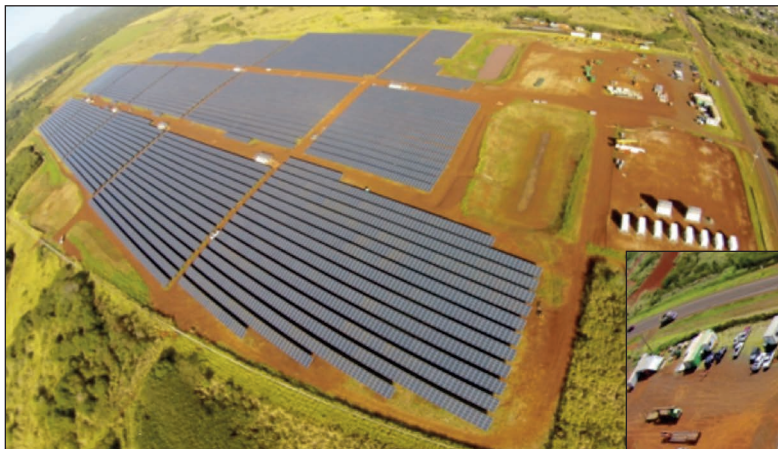
FIGURE 15: Anahola "KRS1" 12 MW, under construction, expected in-service July, 2015
