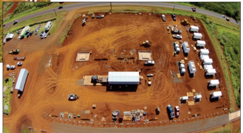
FIGURE 16: Anahola "KRS1" substation under construction, with 6 MW BESS on the right
