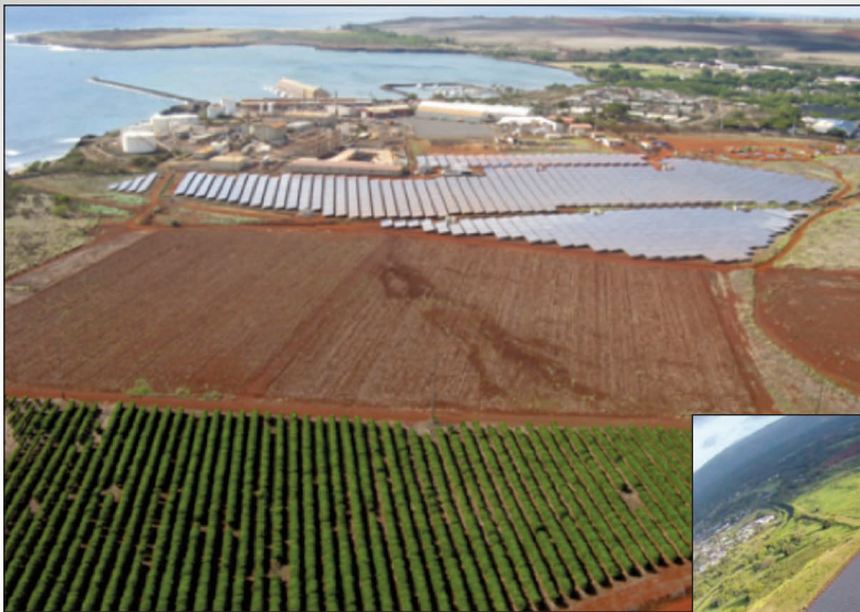
FIGURE 13: Port Allen 6 MW PV, on-line Dec. 2012
