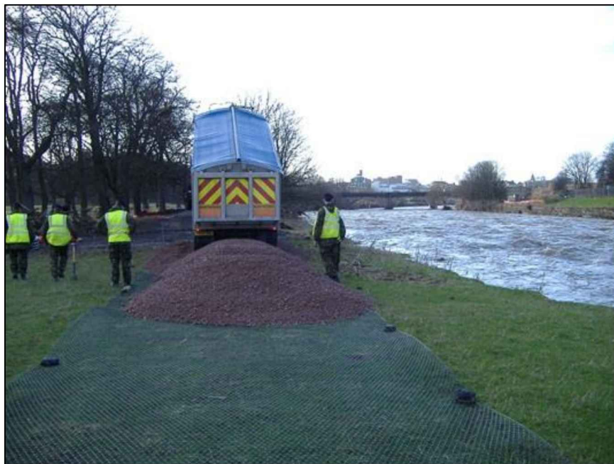
Figure 5-5: Use of Geogrid in Wet Environments (Tensar UK, 2016).
