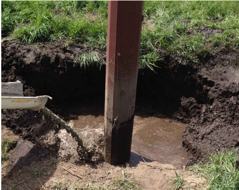
Figure 6-10: Non-uniform Direct Embedment Excavation.
