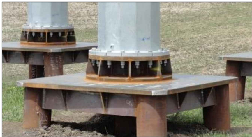
Figure 6-2: Driven Pile Foundation: ATCO Electric Hanna Region Transmission Development Project. (ATCO Electric, 2012)
