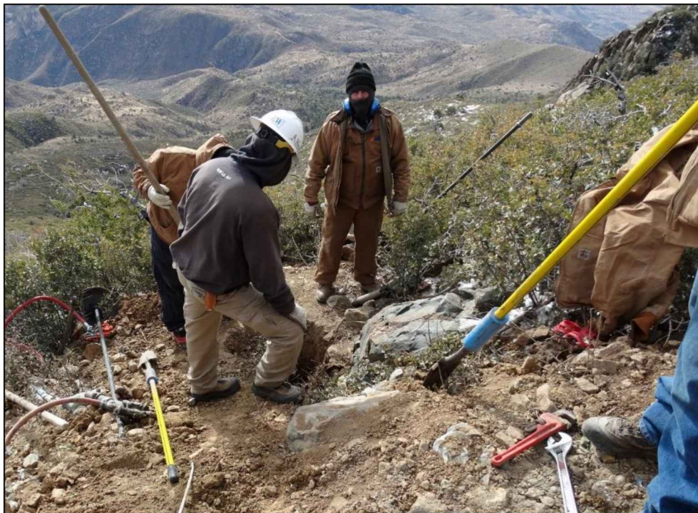
Figure 6-17: Guy Anchor Installation in a Difficult Environment.
