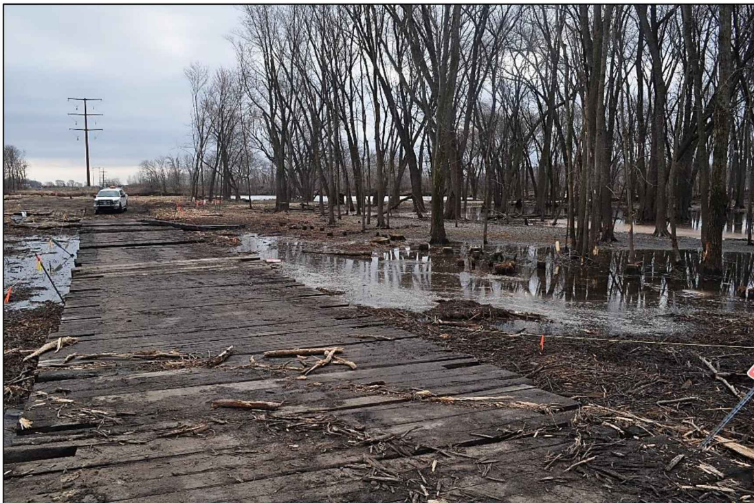
Figure 5-4: Completed Wood Matting Access Road in a Wet Environment.
