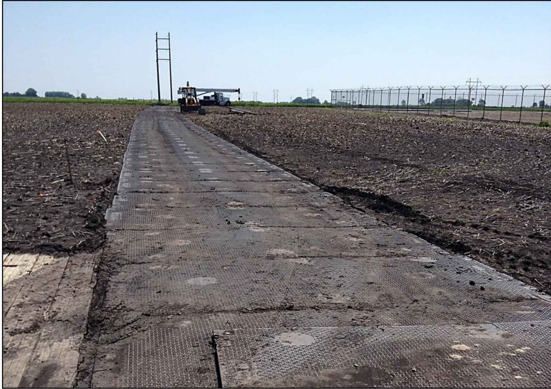
Figure 5-3: HDPE Matting Crossing Farm Field.
