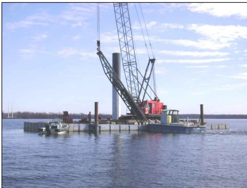
Figure 5-6: Barge in (Stake in Photo) Position to Drive Caisson (Norman et al. 2009).
