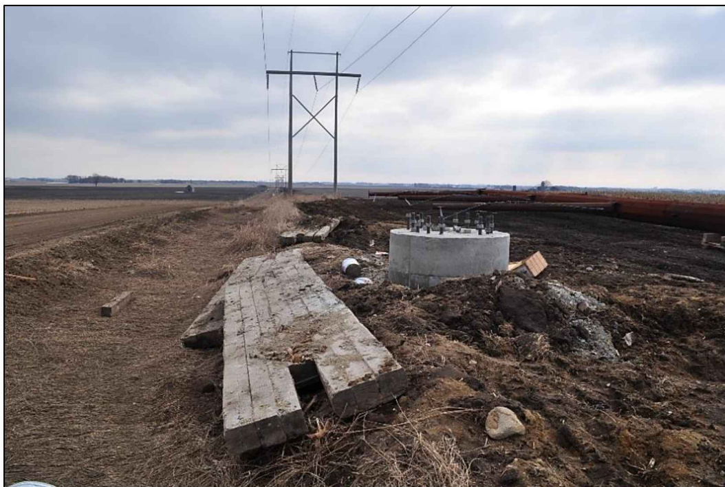
Figure 5-2: Typical Wood Matting for Transmission Line Access.
