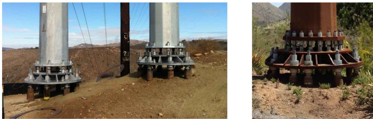
Figure 6-25: Micropile Foundations.
