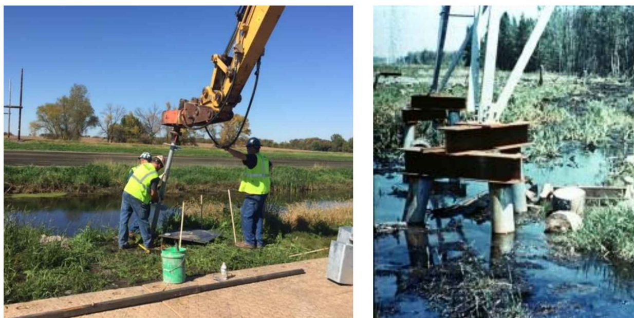
Figure 6-20: Helical Piles Construction (Courtesy Chance/Hubbell Power Systems).
