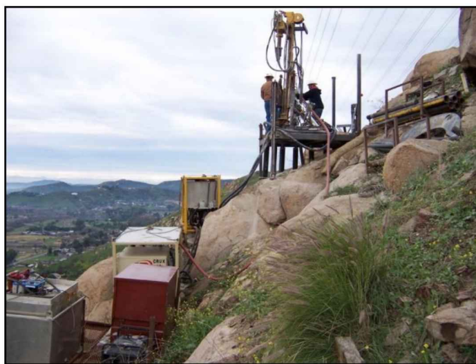
Figure 6-24: Construction of Micropiles. (Photo courtesy of CRUX Subsurface)
