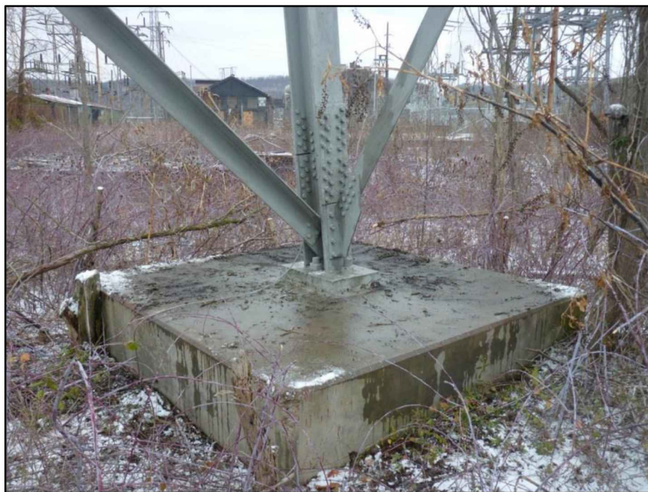
Figure 6-13: Spread Footing Foundation (EPRI, 2012).
