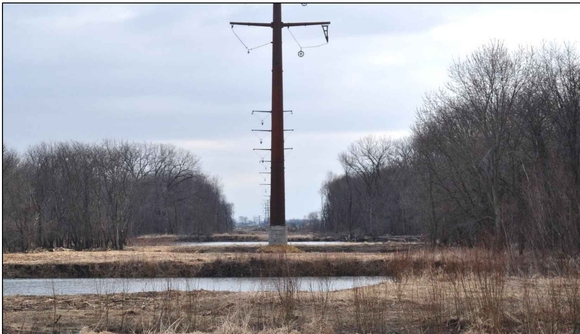
Figure 3-4: Transmission Line located in a Wet Environment (Note high reveal in flood zone).
