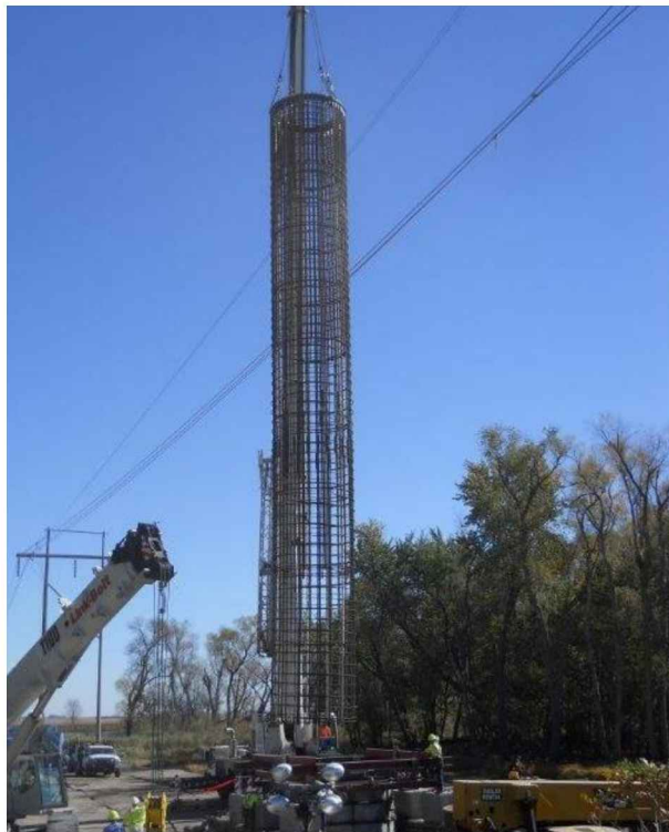
Figure 6-7: Drilled Shaft Construction.
