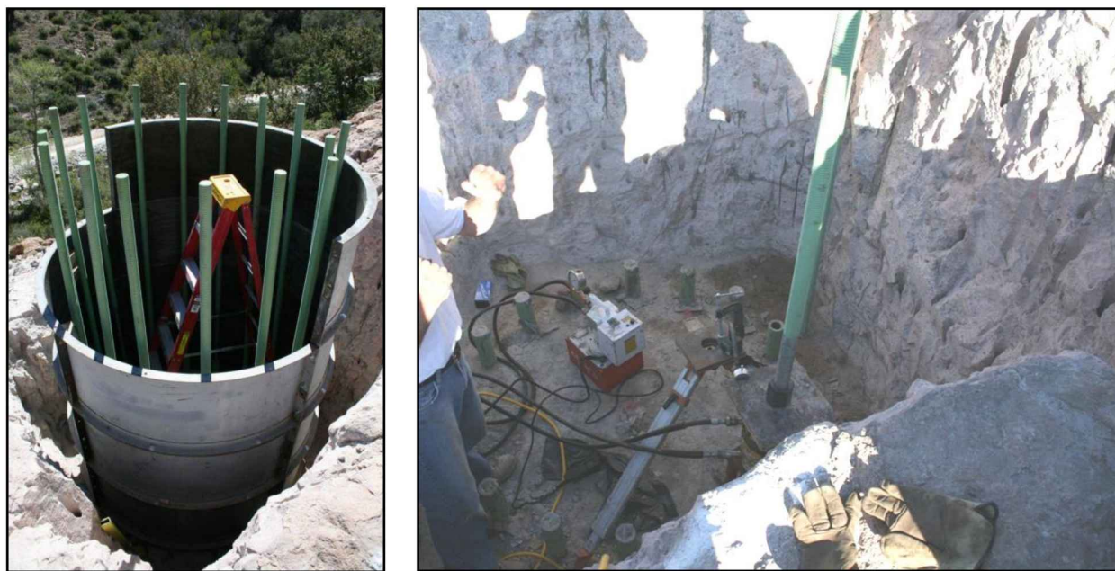
Figure 6-29: Construction of Rock Anchor Foundation.
