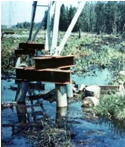
Figure 2 –Helical Pile Tower Foundation
