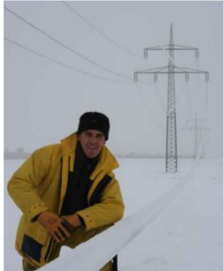
Figure 3-1: Wet snow in Germany, November 2005 (from Cigré TB 344).
