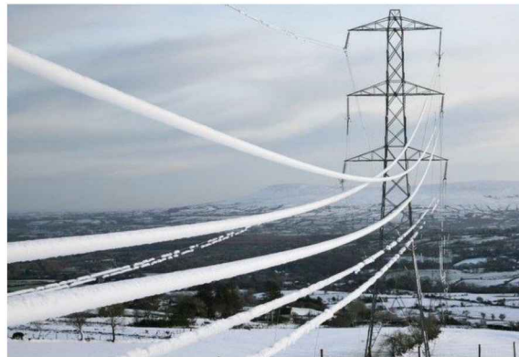
Figure A-1: Wet snow event in Northern Ireland, December 2011. (Source: BBC news)
