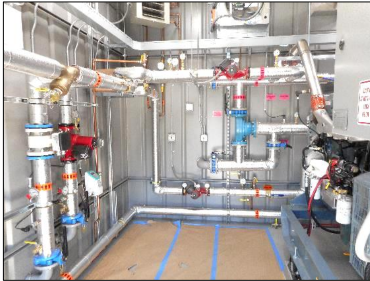
Heat Recovery Piping
