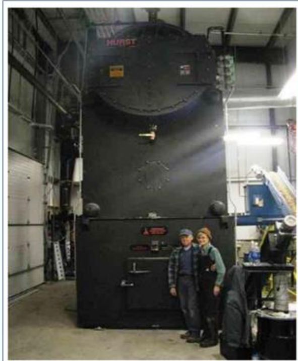
Tok School's biomass-fueled boiler generates 5.5 MMBtu/h, enough to provide steam heat and power for the campus
