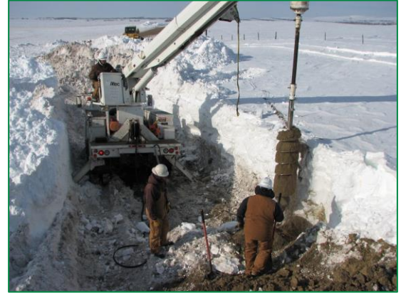
Alliance Co-op Linemen Repairing Damage From 2010 Storm
