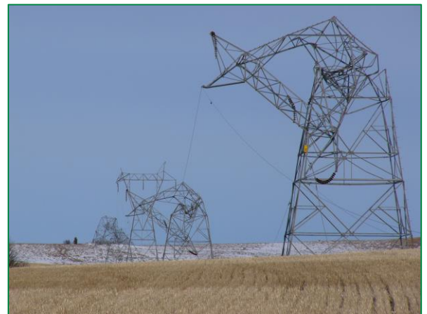
Toppled Towers From 2010 Storm
