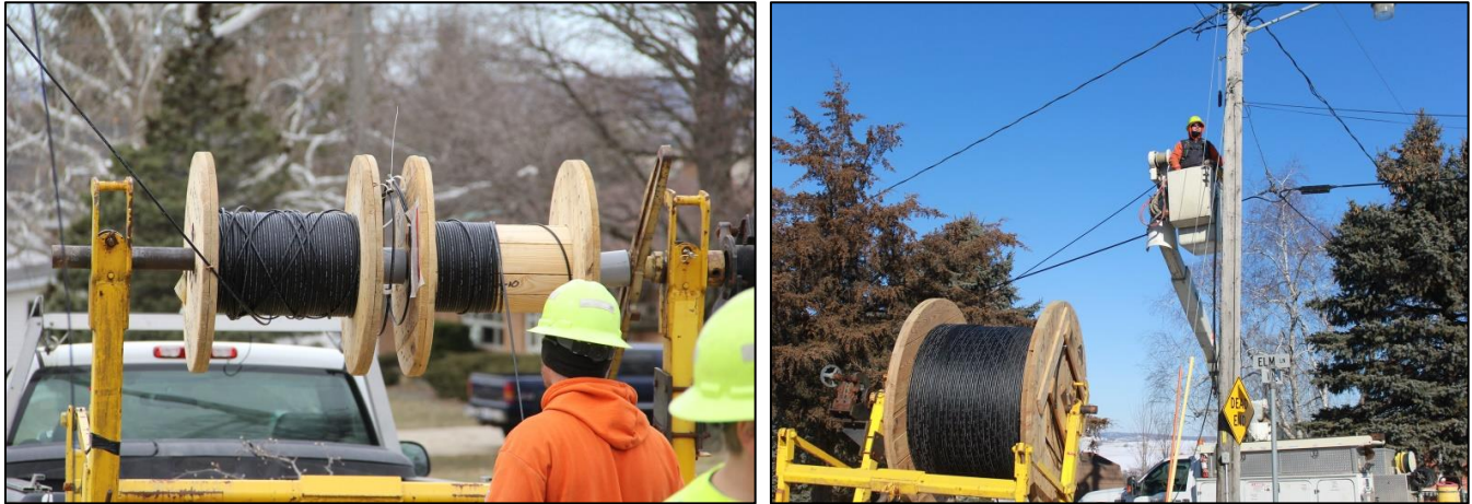
Figure 2. JCE's fiber broadband network under construction. Photos courtesy of JCE.
