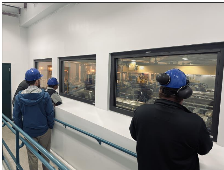
Figure 7: Tour of Southcentral Power Project Energy and Energy Storage Installation
