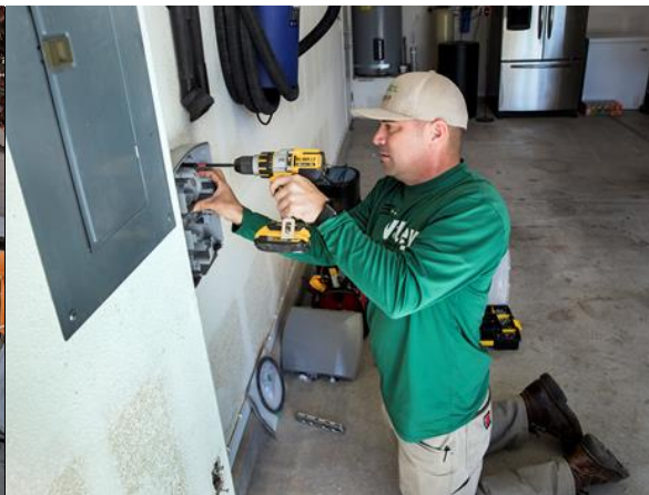
Figure 3. Installing a fiber drop
