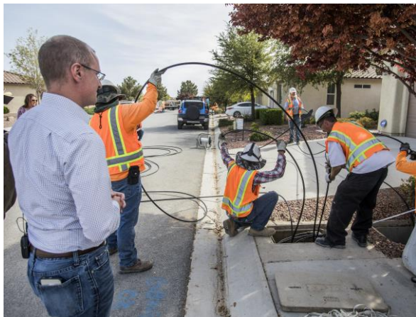
Figure 2. Running underground fiber
