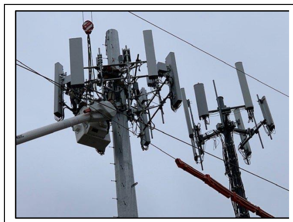
Figure 3. Macrocell site installation. Photo courtesy of RidgeLink, LLC.
