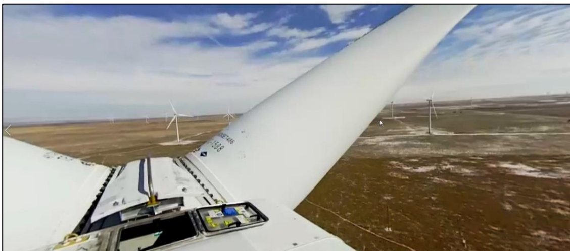
Figure 2. View from top of wind turbine from Tri-State's VR video. Image courtesy of Tri-State.
