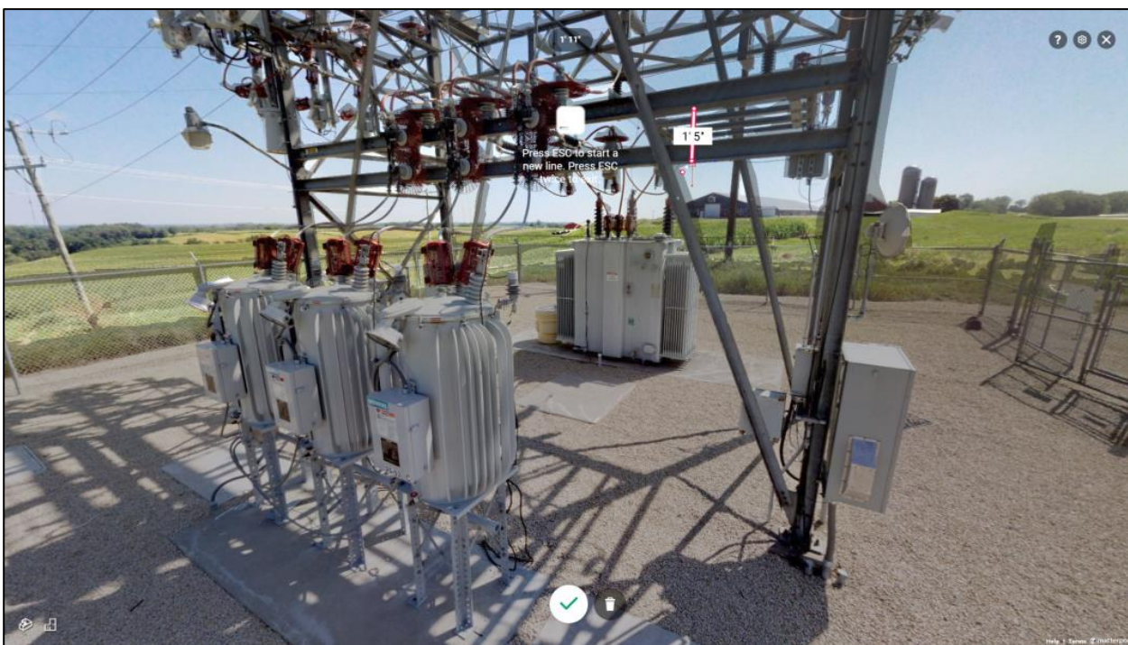
Figure 2. Screenshot of 3D digital scan of a substation, with example dimensions. Image courtesy of Jo-Carroll Energy.
