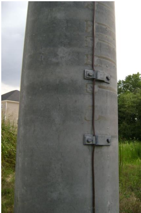
Figure 46: Concrete Pole with Good Ground Connection
