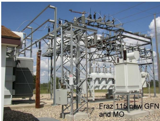
Figure 54: Photo of Ground Fault Neutralizer
