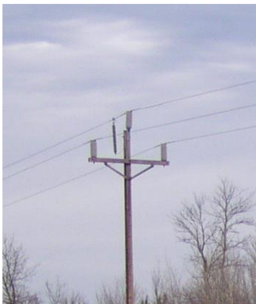
Figure 55: Lightning Arrester on Three-Wire System
