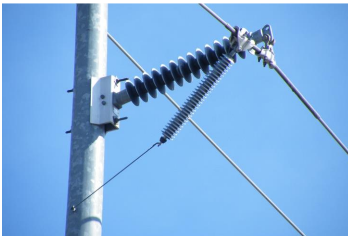
Figure 48: Transmission Line Surge Arrester
