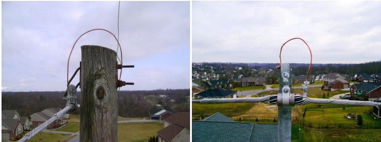
Figure 42: Optical Ground Wire Grounding Connections
