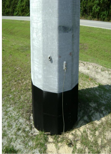
Figure 45: Steel Pole with Good Ground Connection
