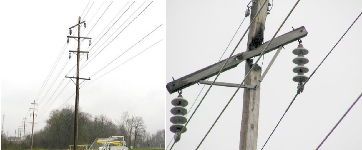
Figure 5: Pole Fire With Close-Up
