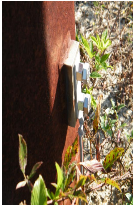
Figure 47: Steel Pole with Good Ground Connection
