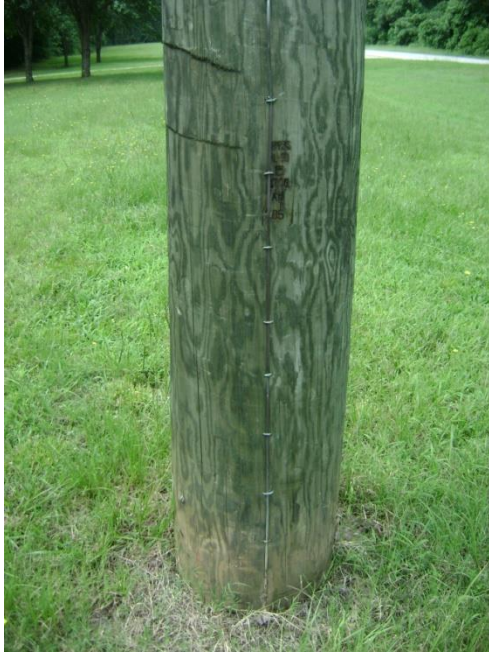
Figure 44: Wooden Pole with Good Ground Connection
